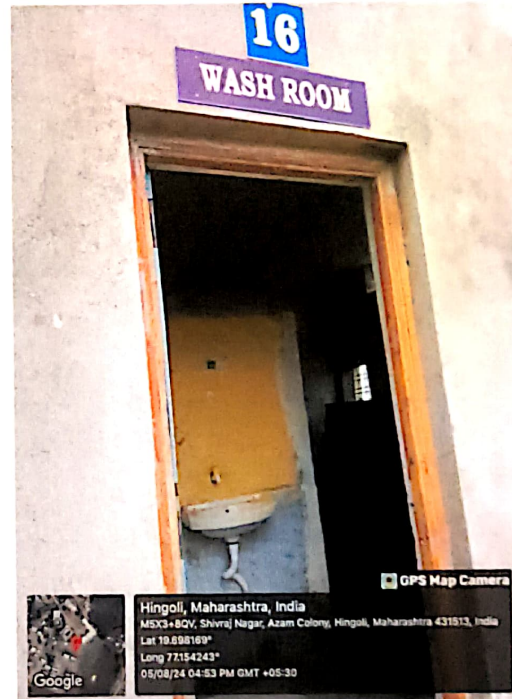
GENTS WASH ROOM
