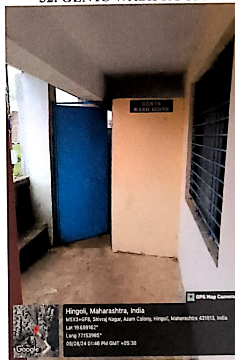
32. GENTS WASH ROOM
