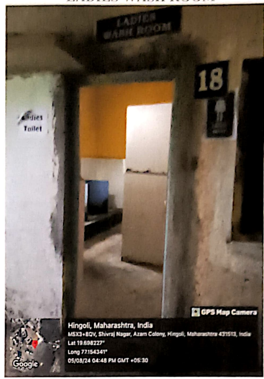
LADIES WASH ROOM
